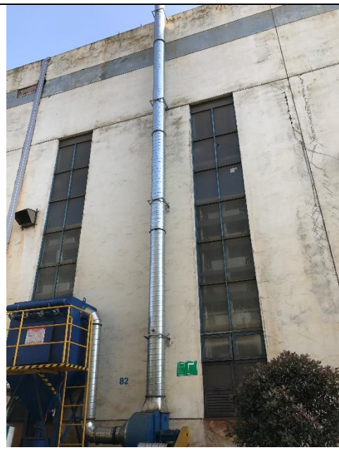
闪光焊处废气排气筒
